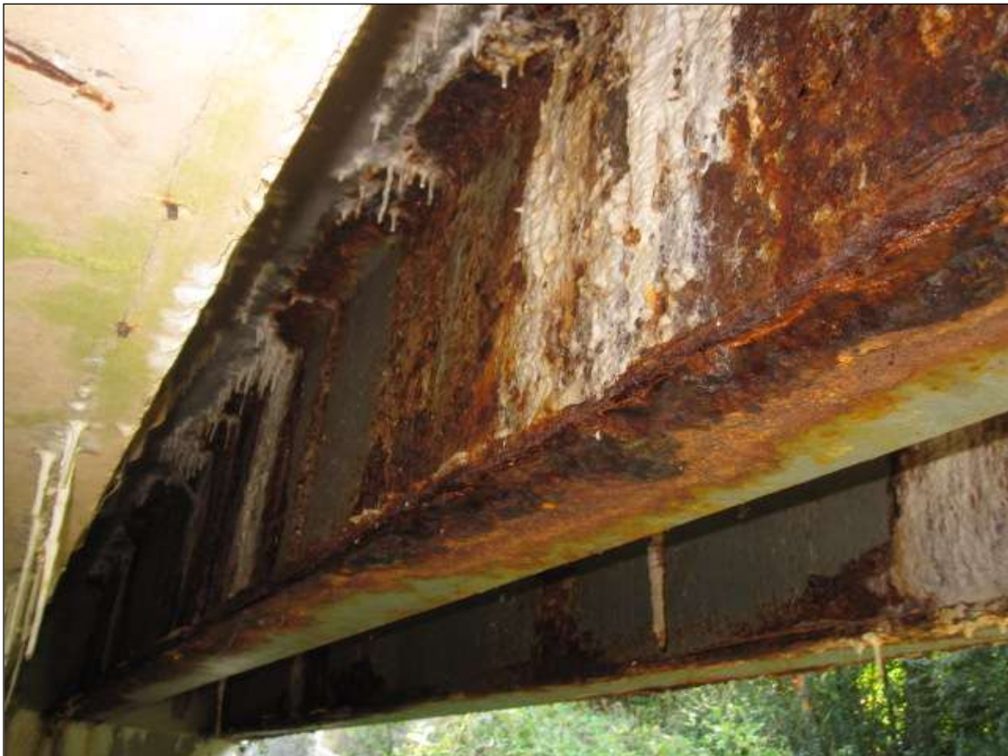
RUST AND CORROSION WITH UP TO 50% SECTION LOSS OF BOTTOM FLANGE BEAM 9 AT MIDSPAN
