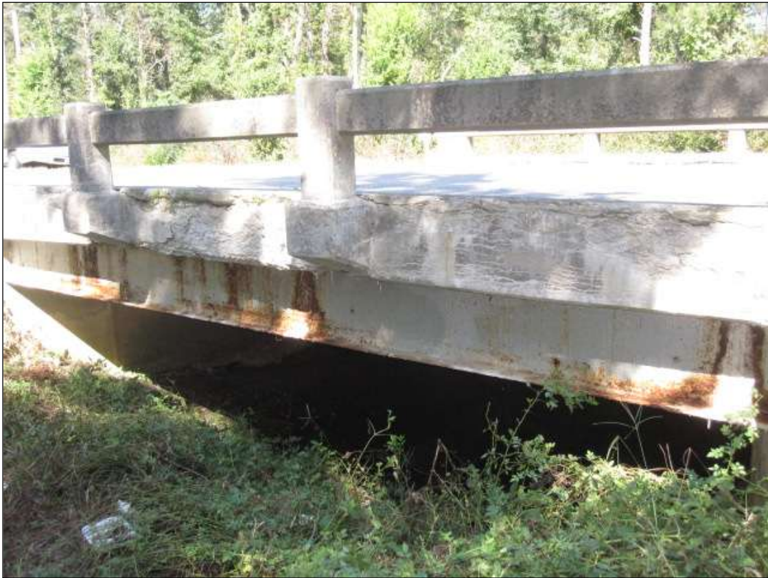
FULL WIDTH X FULL LENGTH SPALLING ALONG EXTERIOR FACE OF SOUTH CURB
