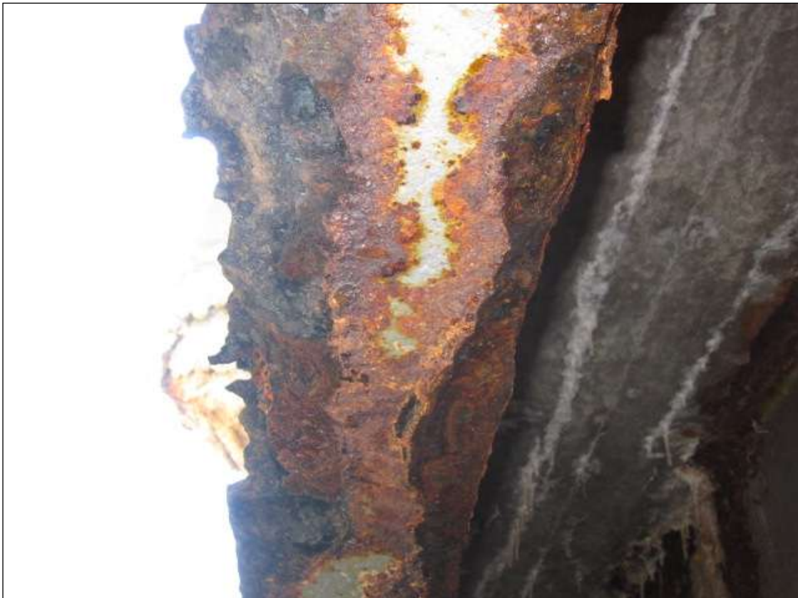
RUST AND CORROSION WITH UP TO 50% SECTION LOSS OF BOTTOM FLANGE BEAM 1 AT MIDSPAN
