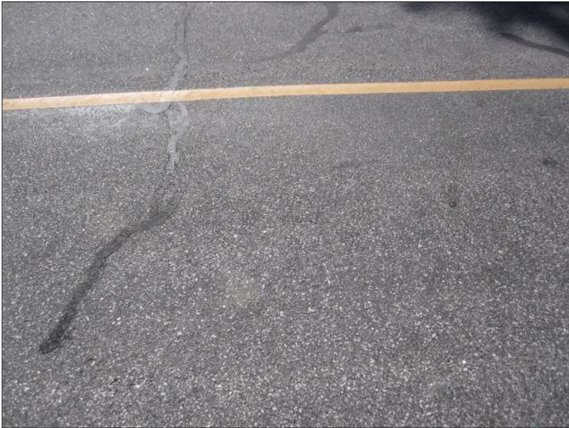
SEALED CRACKS IN APPROACH ROADWAY
