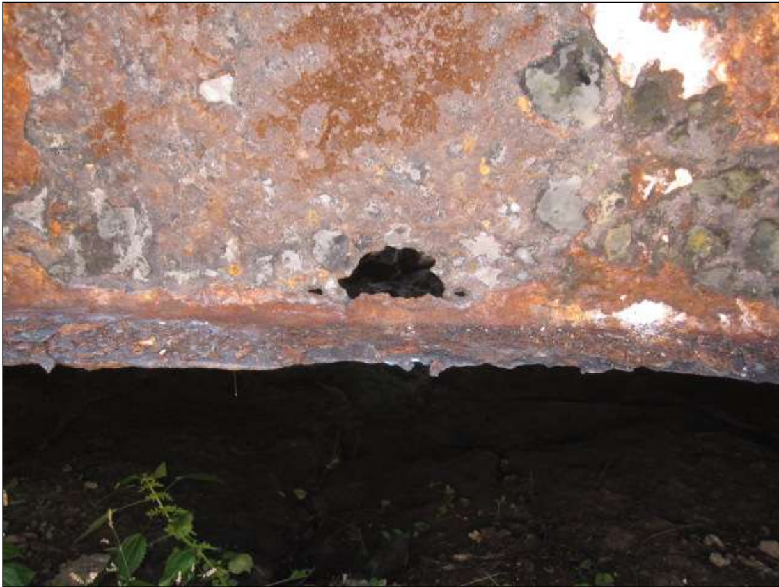
RUST AND CORROSION WITH 5" X 2" HOLE IN WEB OF BEAM 1 AT MIDSPAN
