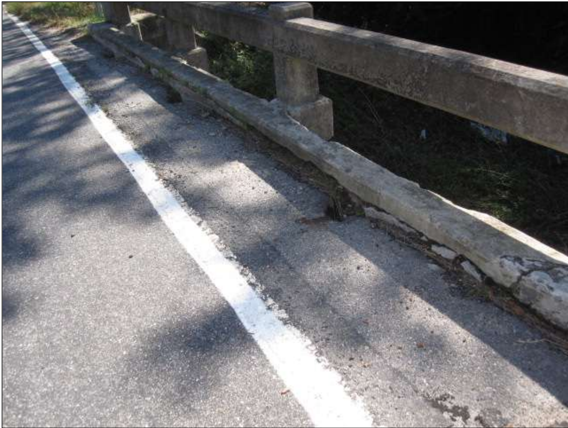
20 FT X 3" X 1" DEEP SPALL IN FACE OF SOUTH CURB
