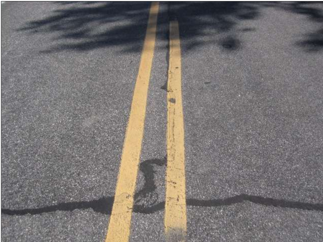
SEALED CRACKS IN ASPHALT WEARING SURFACE
