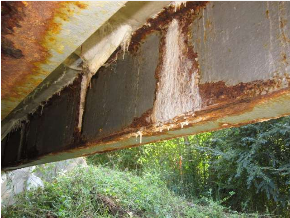
RUST AND CORROSION WITH UP TO 35% SECTION LOSS OF BOTTOM FLANGE BEAM 10 AT MIDSPAN
