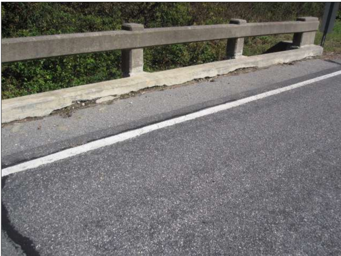
20 FT X 3" X 1" DEEP SPALL IN FACE OF NORTH CURB
