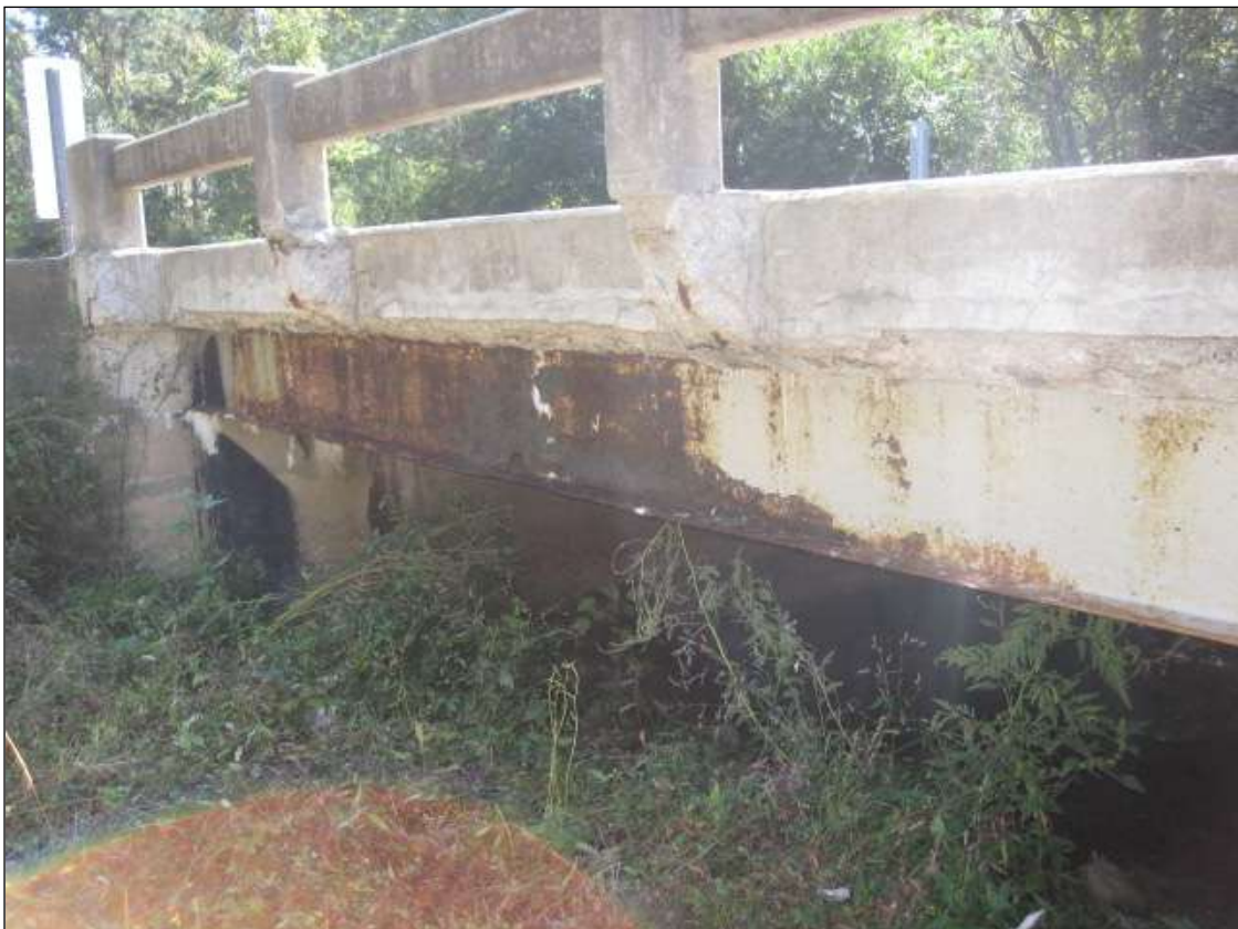
FULL WIDTH X FULL LENGTH SPALLING ALONG NORTH EXTERIOR FACE OF DECK
