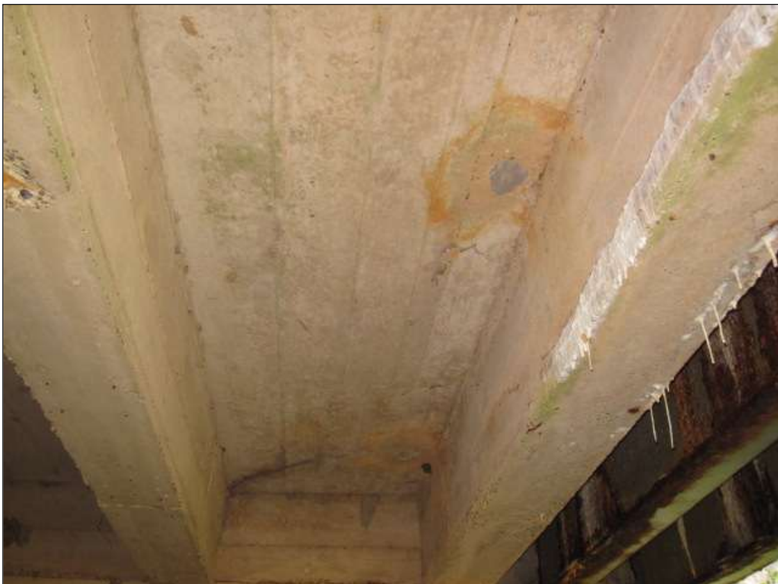
DELAMINATIONS IN BOTTOM OF DECK BAY 7
