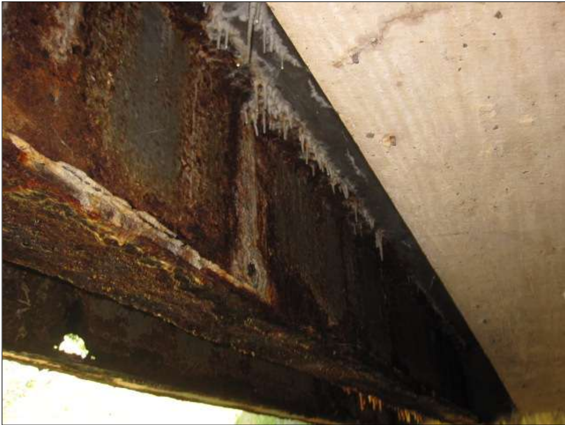
RUST AND CORROSION WITH UP TO 50% SECTION LOSS OF BOTTOM FLANGE BEAM 2 AT MIDSPAN
